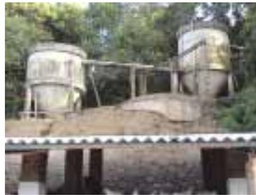
subjected to secondary settling by using another PPS and the sludge at the bottom is re-circulated back. The overflow is sent to stabilisation or polishing ponds comprising three units. The effluents discharged flows to a tree-lined area within the farm, about r 250 metre from the nearest well and over half a kilometer from the river. The discharged water has less than 30 mg/l BOD and is free from E. coli/ coliforms and hence cannot cause any bacterial contamination to the neighbouring wells.
