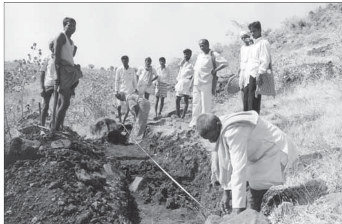
Watershed works in progress: Technical resource persons measure a trench
