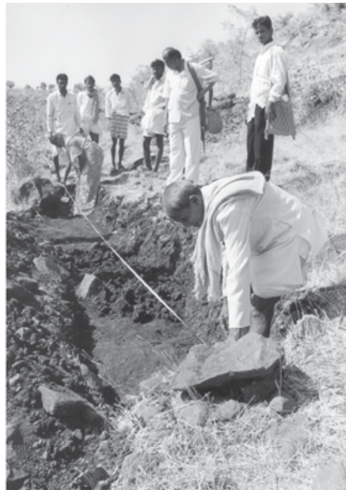
Technical resource persons measure out completed works in Maramuri watershed
